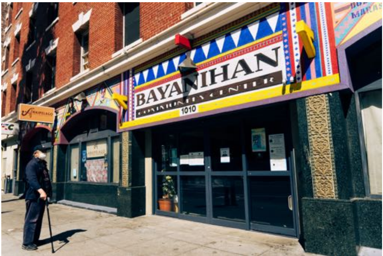
New facade of the Bayanihan Community Center, featuring SOMCAN's Heroes in Our Windows mural, home of Arkipelago Books, the first Filipino bookstore in the United States.
