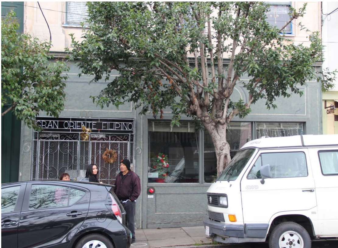
Detail of ground floor façade of Gran Oriente Filipino Hotel, 2017.
